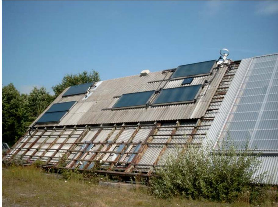
**Figure 3-3: The SDHW test facility. A building with heat storages and control systems is located behind the rack.**
