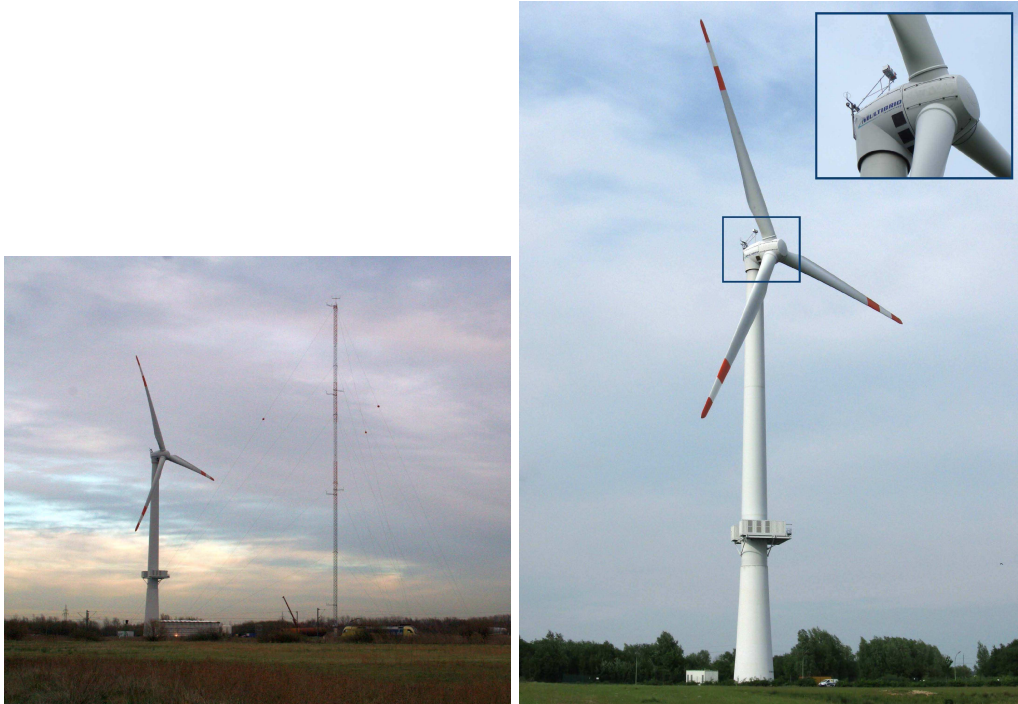
Figure 108: Onshore test site with AREVA M5000 and SWE met mast (102 m) (left) Installation of the lidar system on the nacelle of the turbine (approx. 105 m AGL) (right).
