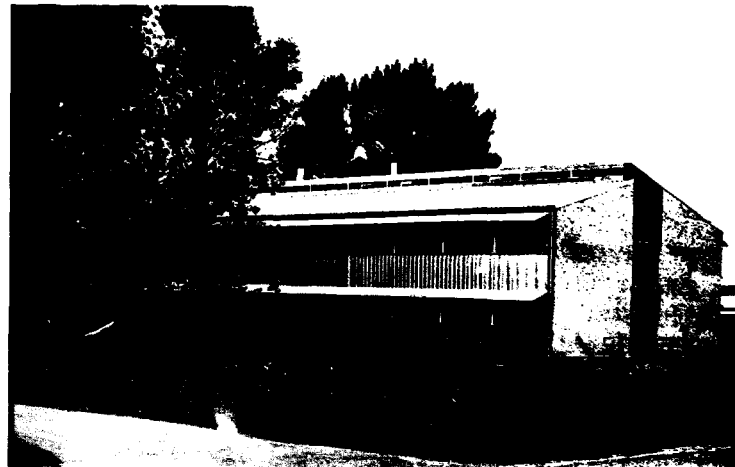
Fig. 9. The extension of the Electronics Department. The Risø standard module, 3 \times 6 \text{ m}^2 , was used for the building.
