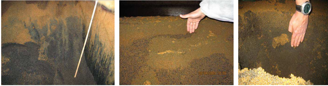
Figure 3.2: Pictures of filter media from rapid sand filters in three different waterworks in Denmark.
