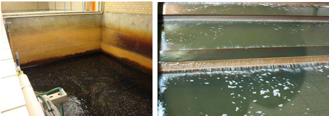
Figure 3.8: Pictures of flow lines in rapid sand filters at two waterworks (from Lopato et al., III).
