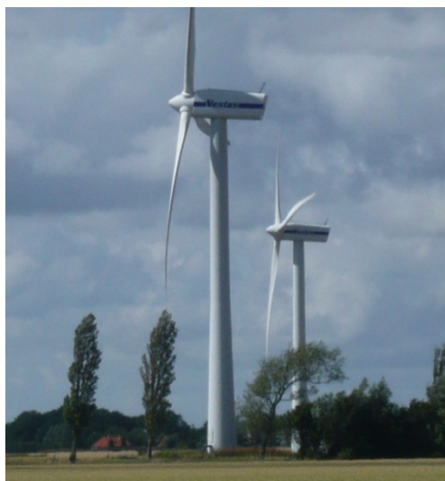
Figure 13.2 Often seen in the landscape: wind turbines that deviate significantly in yawing direction
