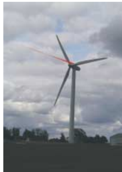
Figure 16 Laser anemometer being used on wind turbine nacelle for control and power performance verification purposes (Re. Rene Skov Hansen, Risø)
