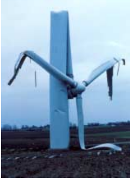
Figure 7 Safety and structural integrity are important in the design and detailed testing is a necessity
