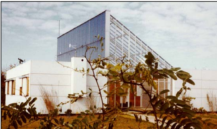
Zero-Energy House at the northern area of DTU.
