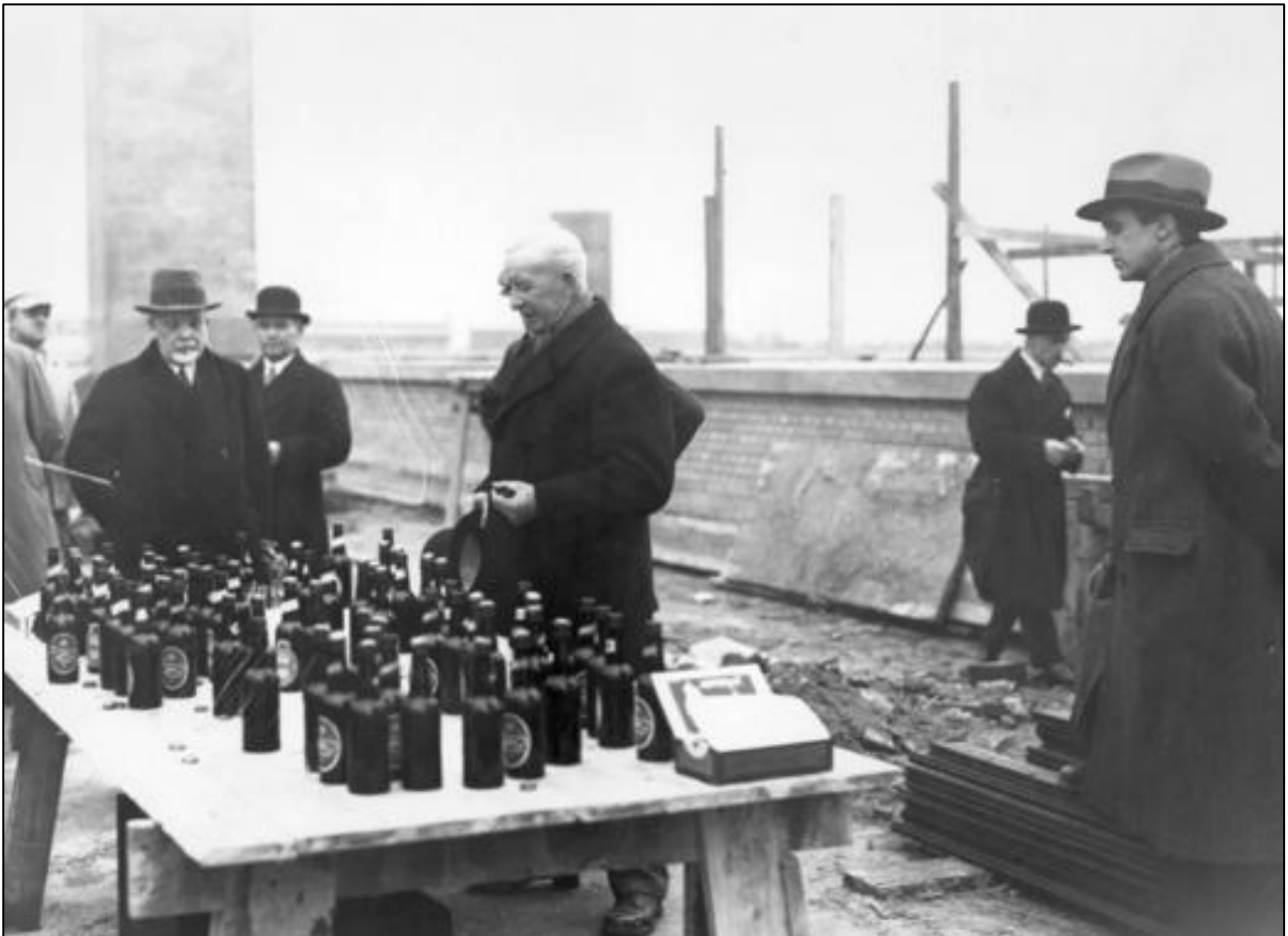
Laying of the foundation stone for the building work at Østervoldgade in 1929. The rector P. O. Pedersen stands at the end of the table.
