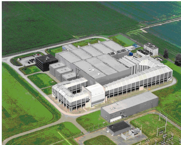
Figure 4.1 LLF (Large Scale Low Speed Facility) of DNW (German Dutch Wind Tunnels) (Picture from http://www.twanetwerk.nl )
