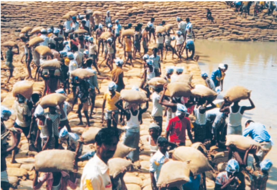
Figure 4.16: Closure dam under construction at Jamuna river, Bangladesh
