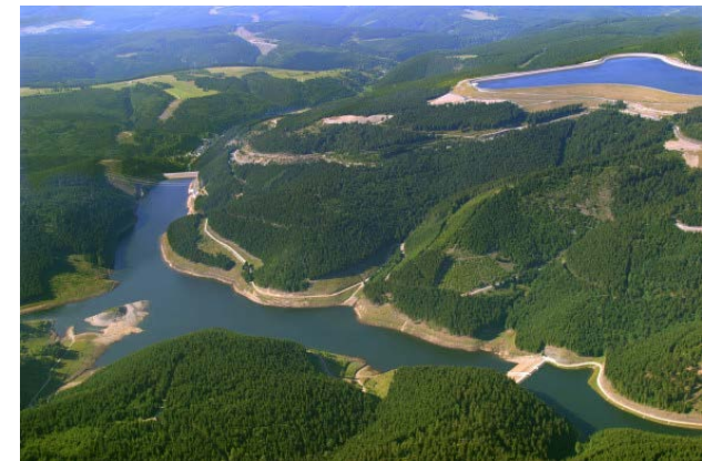
Vattenfall 1060 MW PHS plant in Goldisthal, Germany
