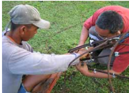
Re-tensioning of guy wires and tightening of nuts
