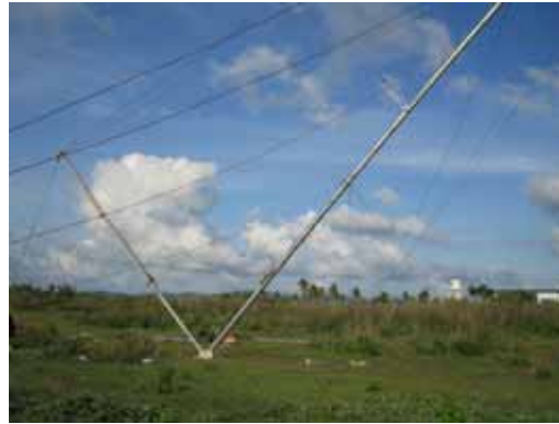
Tower raised 45 degrees from ground level
