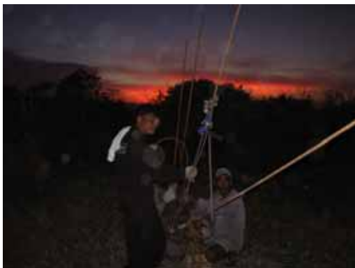
Straightening of the tower and tensioning of the guy wires
