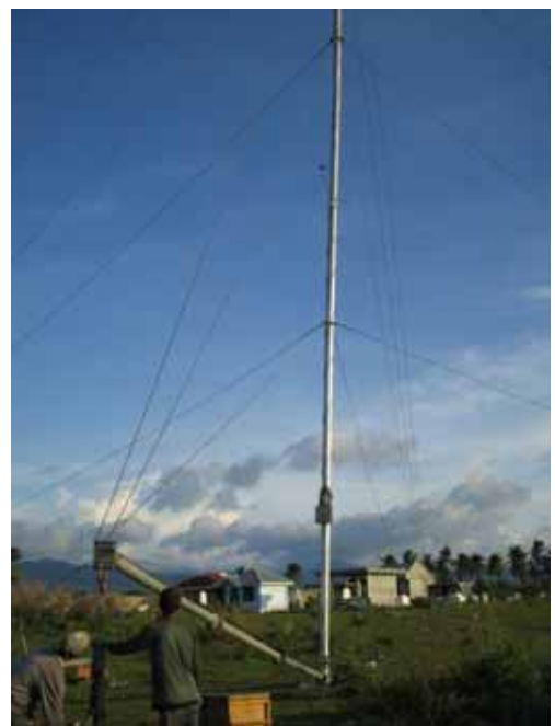
Tower almost erected
