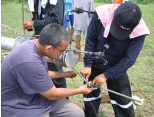
Installing the lightning arrester and grounding
