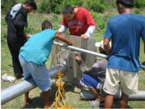
Fastening the tower to the base plate
