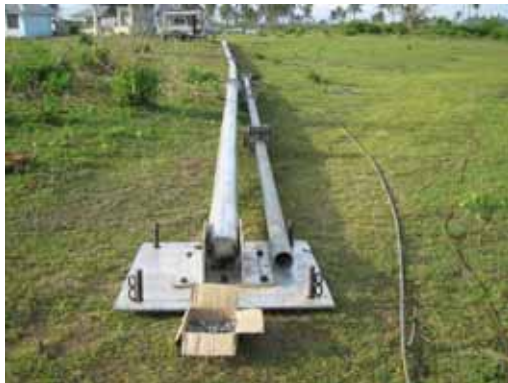
Assembling the gin pole
