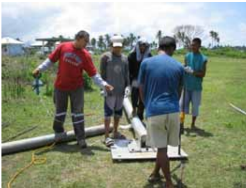
Measuring Anchor Placements
