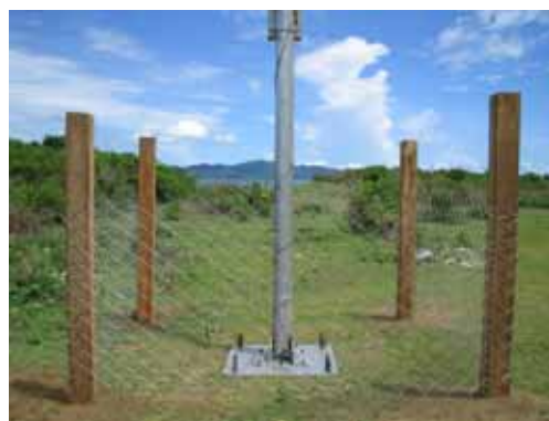
Construction of security fence around the tower
