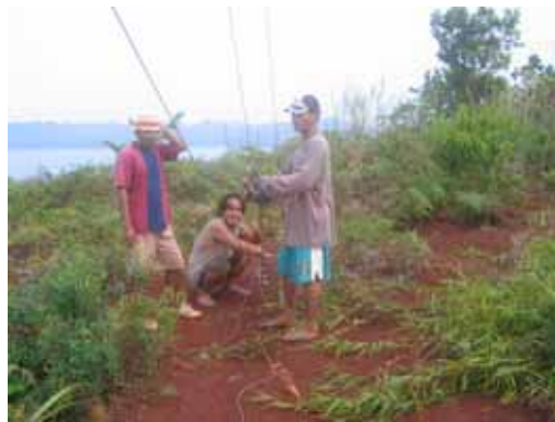
Adjusting the tension of Guy Wires
