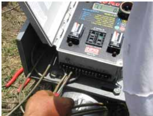
Connecting instrument cables to the logger
