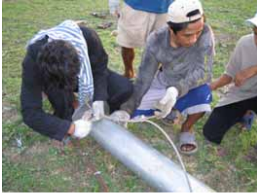
Fastening the Guy Wires
