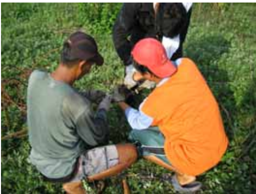
Guy wires placed at respective anchors
