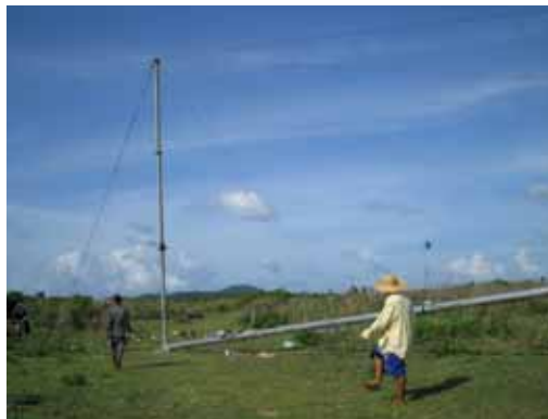
Raising-up the tower
