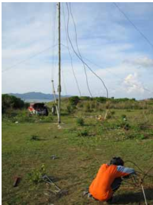
Adjusting the guy wires tension
