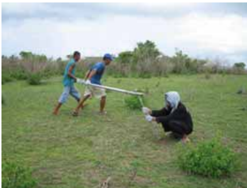
Drilling of Anchors
