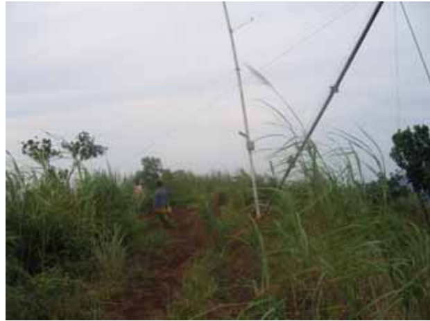
Erecting the 30-meter Tower
