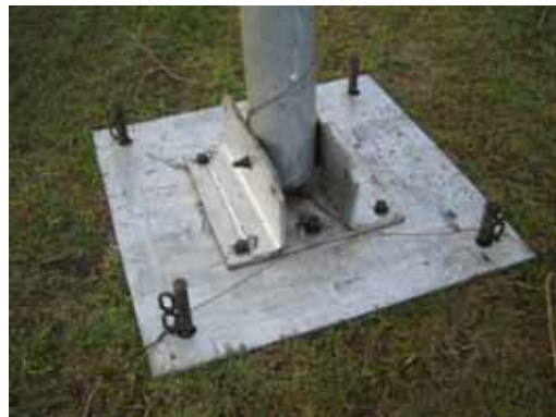
Grounding wires
