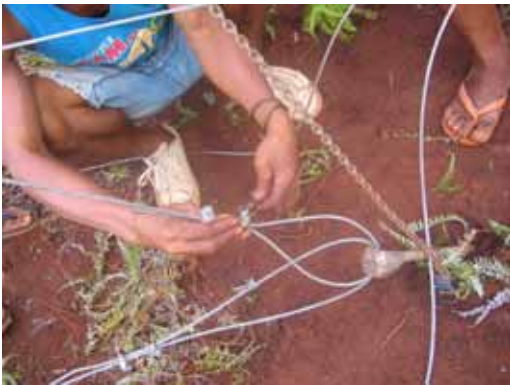
Adjusting the tension of Guy Wires
