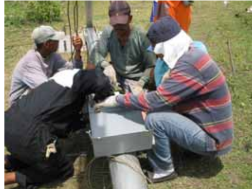
Installing the data logger shelter box
