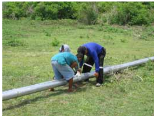
Assembling the Tower Segments
