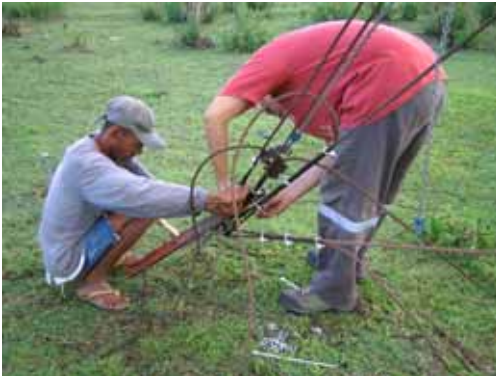
Re-tensioning of guy wires and tightening of nuts
