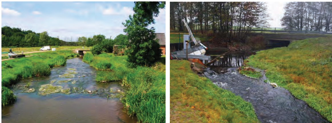
Figure 8. Bypass water passage at Løjstrup Trout Farm (left) and at Bregnholm Mølle Trout Farm with inlet and grids (right). Photo: Lisbeth J. Plesner.
