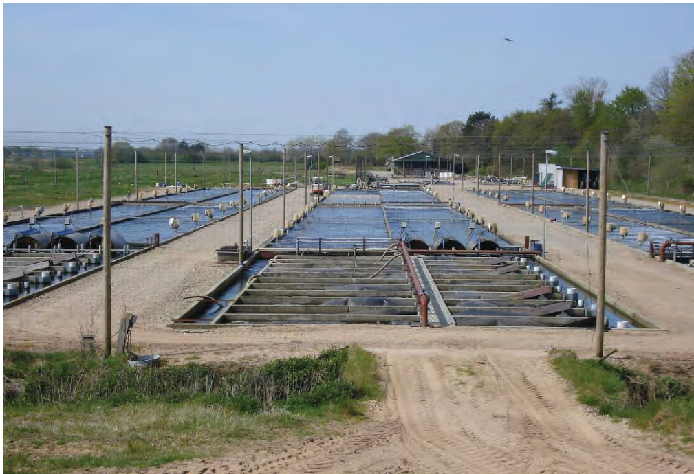
Figure 14. Kongeåens Model Trout Farm (type 3). The production units include three sections, each consisting of two concrete raceways with micro sieves (mesh size 74 µm) in front of the biofilter sections (foreground). In the background to the left, the plant lagoons consisting of the former earthen ponds and the inlet and outlet channels are visible (Svendsen et al., 2008). Photo: Lars M. Svendsen.
