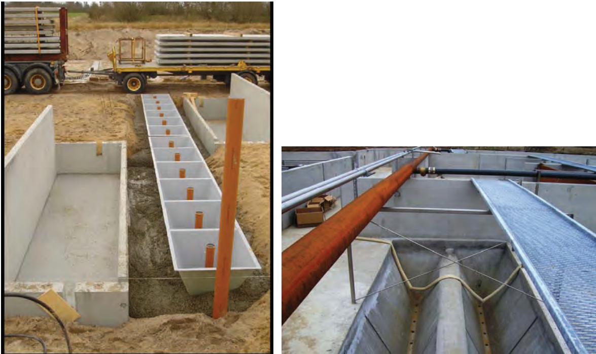
Figure 17. Sludge cones are mounted at the downstream end of each raceway section across the full width of the raceway and in line with the raceway bottom. To the left, each raceway has six separate sludge cones, whereas the raceway to the right has one sludge drain along its full length, with only one discharge outlet.
