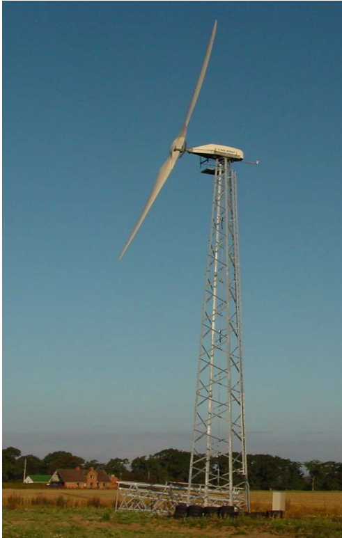
Figure 2 Gaia Wind 11kW wind turbine
