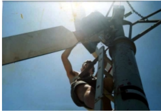
Installing a 2.5 kW windturbine for remote area power supply in Africa
