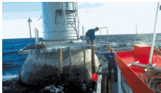
Figure 1. Repair works at Tunø knob Wind Turbine Site (Photo: Elsam)
