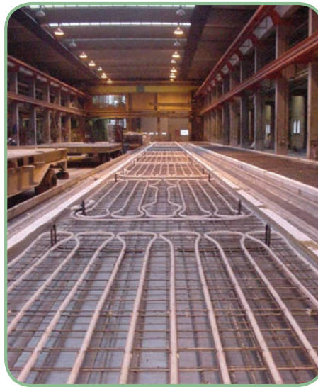
Photo 1: Prefabrication of slabs with integrated piping.
