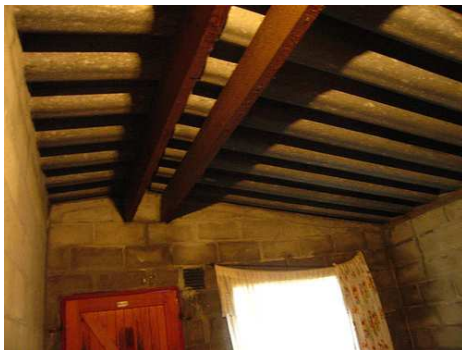
House before intervention showing uninsulated roof and cement brick walls.
