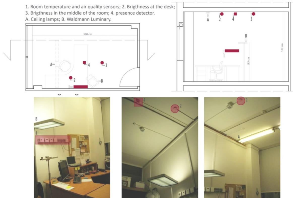
Figure 1. Installed sensors in office rooms.
